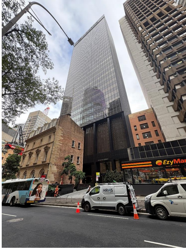
Figure 1: 25 Bligh Street Sydney, viewed from the east.
